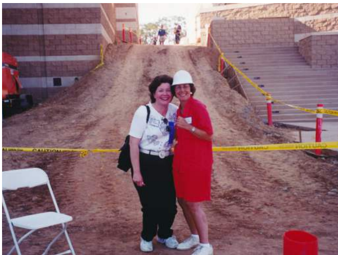
Excitement abounded as Beth Israel members and staff watched the sloping dirt lot become a five-building, Jerusalem-inspired campus.
